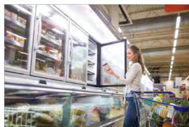
Super Market Refrigeration
